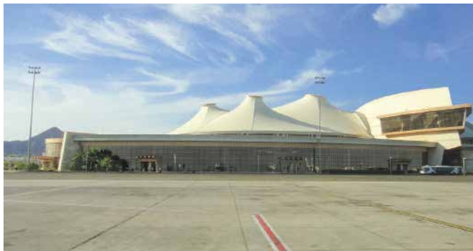
SHARM ELSHEIKH AIRPORT Power
