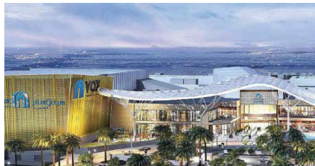
THE ALMAZA MALL ALFUTTAIM GROUP Cable Trays
