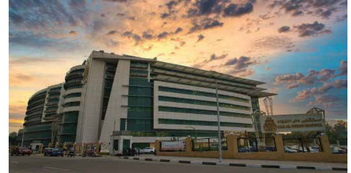
DAR EL FOUAD HOSPITAL Bus Trunking System
