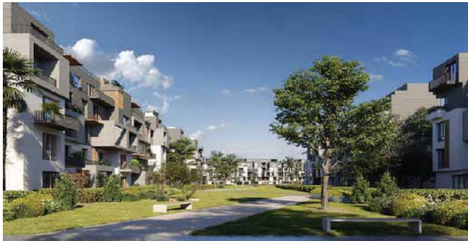
SODIC-EAST-NEW-CAIRO-COMPOUND Lighting Poles
