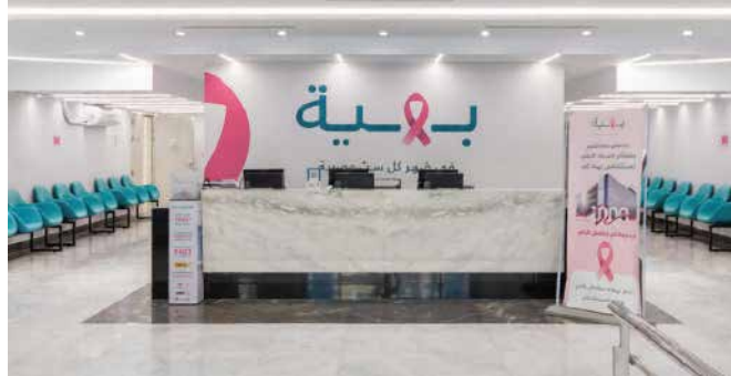
BAHEYA HOSPITAL Cable Trays + Facade + Indoor Lighting
